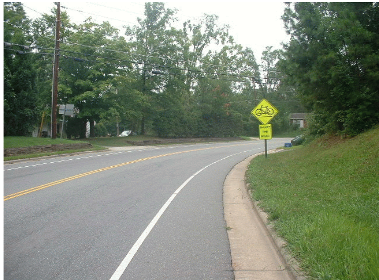
Figure 2. The “Share The Road” sign used on a low speed, low volume street with a bike lane is a misuse of the warning sign. S. Greensboro St., Carrboro, NC.
