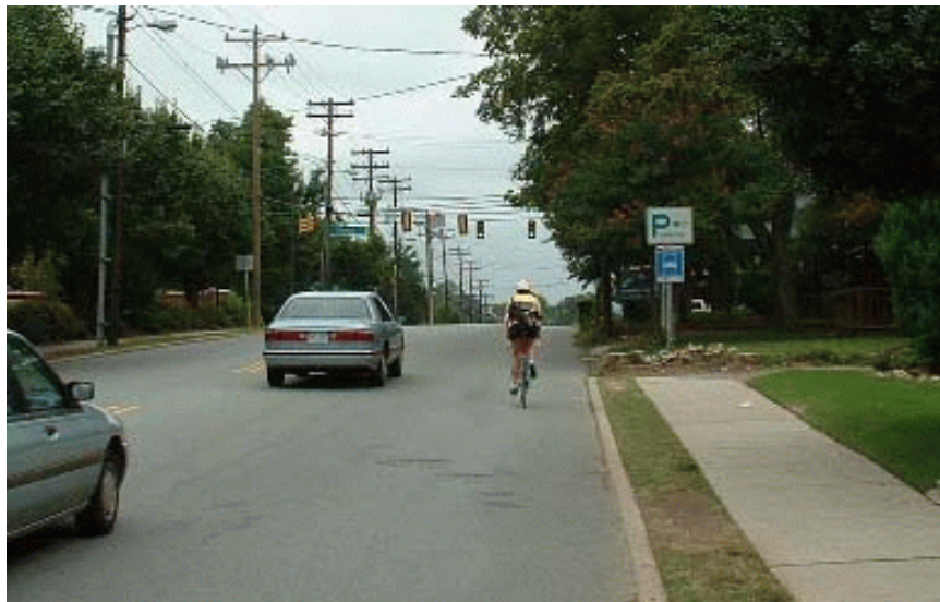
Figure 3. A 16 foot WOL is the same width as a typical BL road.
