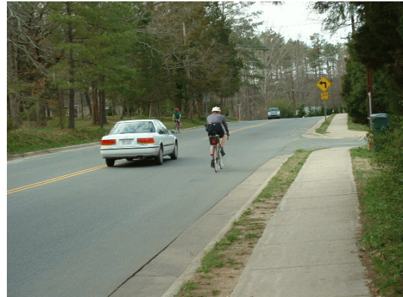
Figure 2. A 16 ft WOL, BL stripe removed.
