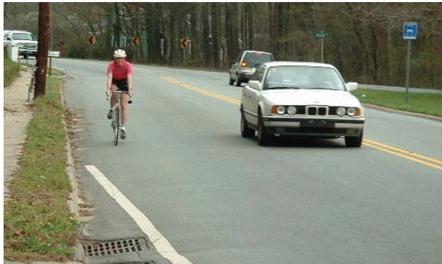
Figure 5. In a 15-foot lane (grate edge to centerline in this case), bicyclists have zero negative impact on roadway capacity.
