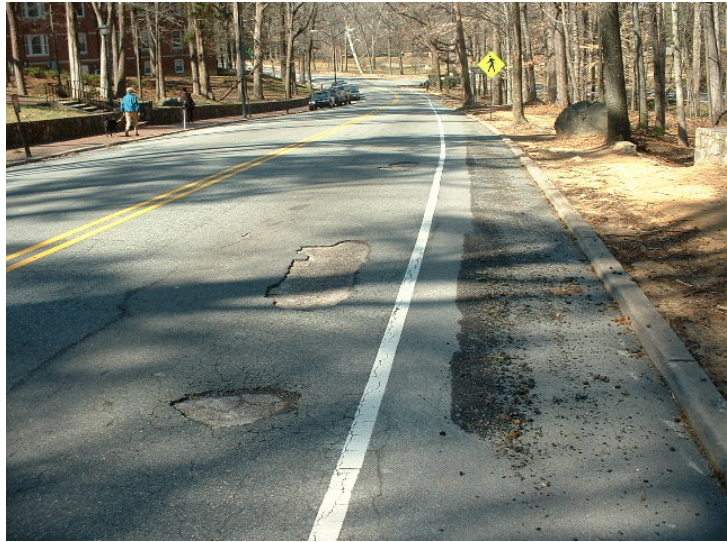
Figure 2. Motor vehicles sweep debris right, just over bike lane stripes to where they don't operate, causing bicyclists to ride further left. Without the stripe, debris is pushed further right, out of bicyclists' typical traveled way. Country Club Rd., Chapel Hill, NC.
