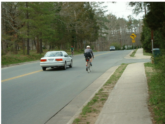
Figure 4. A 16 ft WCL. The bicyclist can use as much or as little of the lane as required. Motorists can easily overtake.
